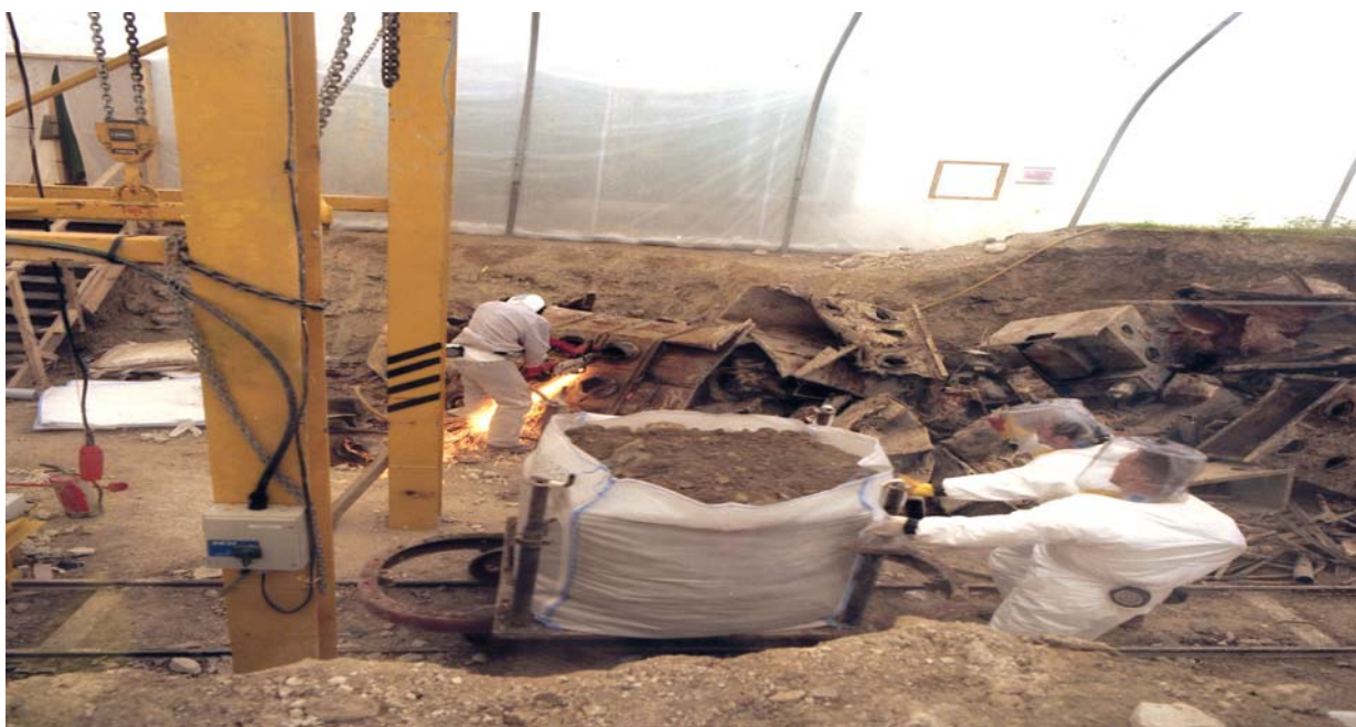
Figure 2.2: Remediation of Contaminated Land
